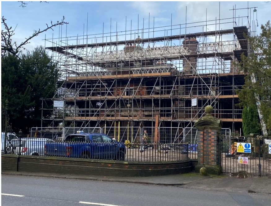
Betley Court scaffolding, January 2021
