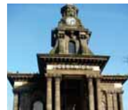
5 Ceramica's buildings form key landmarks and focal point.
