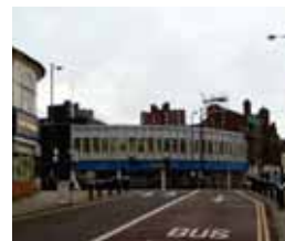
4 Poor quality buildings occupy key landmark locations and add little positive character to Stoke.
