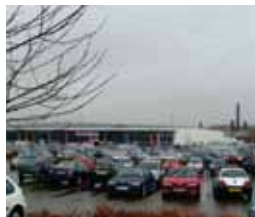
4 Surface car parks provide for the needs of visitors, but are generally designed to serve a particular development rather than the centre as a whole. Some appear fragmented and impact negatively on the townscape.
