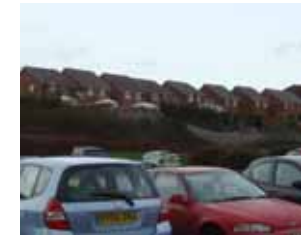
This recent development does not relate well to the existing topography and creates a poor edge along the slope.
