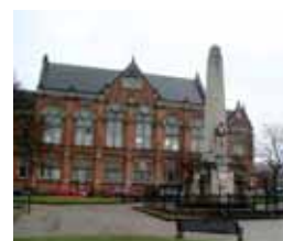
3 The Courts building and Albert Square create a distinctive, high quality place. However it is not visible from the main traffic thoroughfare and people passing may not be aware of it.
