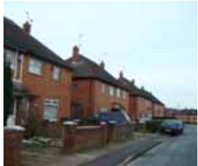
The quality of this housing typology depends on the original built quality and state of maintenance.
