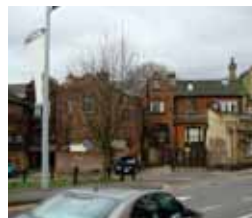
5 Although in terms of massing, enclosure and street alignment the approach is positive. It is let down by the rear elevations of development along St. Peter's Close, which terminate the vista.
