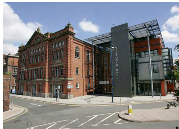
Figure 9.4: Victoria Hall, City Centre - The extension to the listed building provided new facilities that allowed the hall to continue to have a viable use into the future. These were provided in a new building which leaves the historic building intact and its historic fabric largely undisturbed. The design of the extension relates well to the height, bulk and scale of the original building and is set back from the line of its frontage. It is clearly a contemporary building although it uses a typical local material, terracotta
