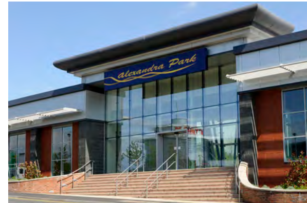
Figure 2.22: An example of good design practice within the region - Scotia Road, Tunstall, where the design evolved through a process of pre-application design review to address the street frontage and create a high quality public realm both on the street frontage and within the site
