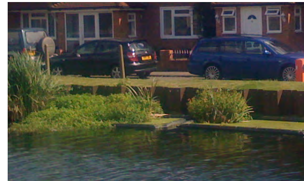
Figure 6.13: Swimming planters create the opportunity to re-naturalise the river/canal edge, enhancing both its appearance and biodiversity
