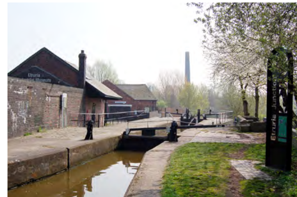
Figure 6.14: Etruria Industrial Museum - a traditional approach to the canal side and towpath
