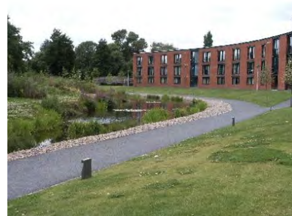
Figure 11.16: Jubilee Campus, Nottingham - University buildings set around a lake and wetlands, which manage surface water run-off and contribute to cooling of the buildings, so playing an important role in the environmental performance of the building as well as creating an attractive setting and outlook for the occupiers
