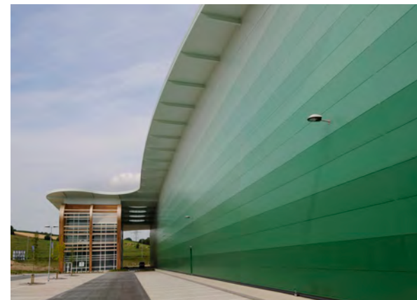
Figure 8.7: Blue Planet, large scale carbon positive industrial development that uses a sculptural form and a gradation in colour on its elevations to make sure it sits well in its surroundings. All of its energy and heat comes from renewable sources and its drainage is sustainable, with rainwater harvesting and controlling of surface water run-off on site, using a series of ponds which have been landscaped to enhance local ecology and to create areas with public access
