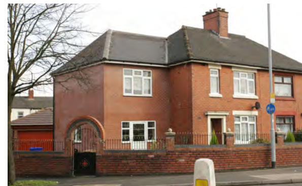
Figure 7.26: Smallthorne, an example of an extension at the same scale as the original building but set back from its frontage, which continues its materials and key details
