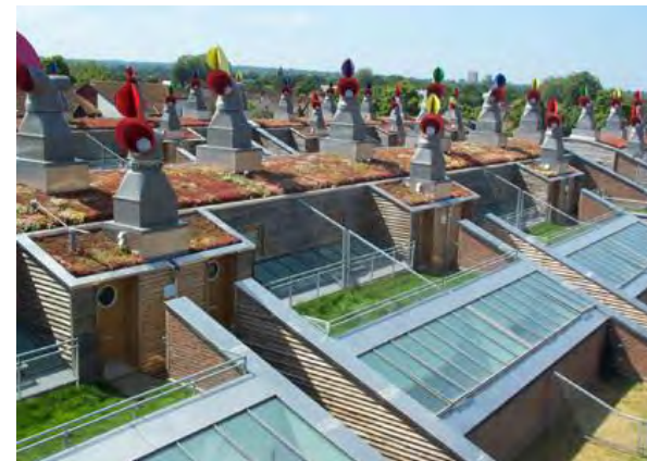
Figure 2.17: Bedzed, Hackbridge - green roofs contribute to surface water management and provide garden spaces for all residents and can help to create a 'green' setting in areas that are viewed from higher ground
