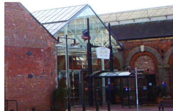
Figure 4.23: In Swindon, historic industrial buildings have been converted into a successful outlet shopping centre and visitor attraction. The role identified for Stoke includes ceramics factory shopping
