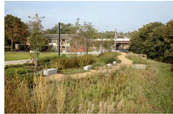
Figure 2.16: River Quaggy, Lewisham - One component of a project to re-naturalise the river, removing concrete culverting in parks and open spaces and creating wetlands. This not only enhances the open spaces but also helps to reduce the risk of properties flooding by creating areas of new floodplain
