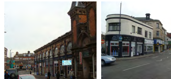
Figure 4.18: There is a variety of materials in the town centre, with the Market (left) in brick with stone decoration and buildings on Market Street (right) in render and stone
