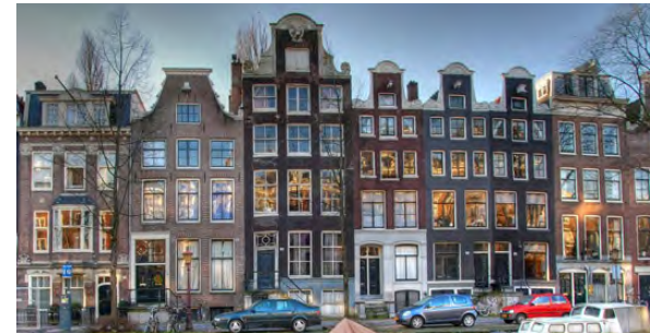
Figure 7.16: Example of Amsterdam, individual buildings vary, but a consistent character is achieved as all use the same material, similar window proportions have a vertical rhythm
