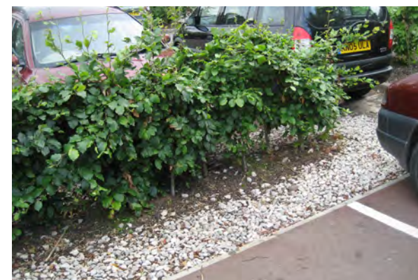
Figure 8.10: Gravel filled swale is part of sustainable drainage and allows planting to be incorporated into parking areas development.
