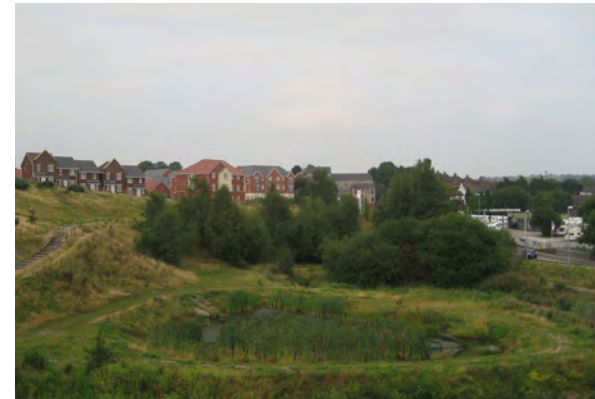
Figure 11.18: A SUDS feature near Sneyd Green, where the balancing pond, creates a wetland landscape and helps add to the biodiversity of the landscape
