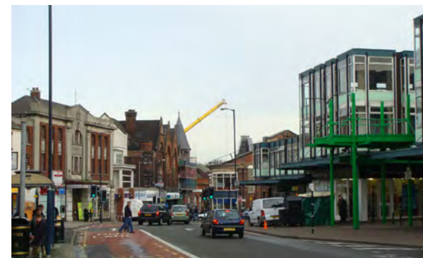
Figure 4.19: The 1960s shopping precinct is occupied, but would benefit from refurbishment to create a stronger sense of place
