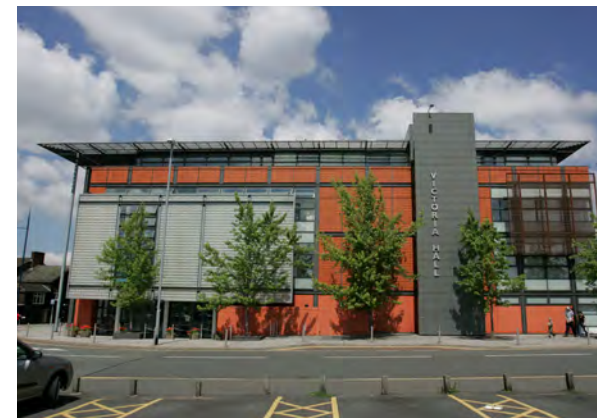
Figure 4.7: Victoria Hall, an example of the contemporary use of local materials, in this case terracotta cladding, relating the building to its City Centre context. Although the building is large, the elevation has a human scale that fits into the City Centre
