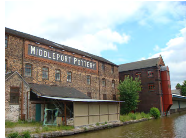
Figure 6.10: Middleport - former pottery buildings in this area present a potential opportunity to create a canal-side destination that draws visitors and local people to enjoy the waterfront location
