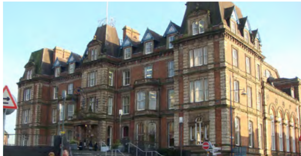
Figure 1.6: Victorian use of traditional local materials at Hanley Town Hall - red brick, buff brick and buff sandstone
