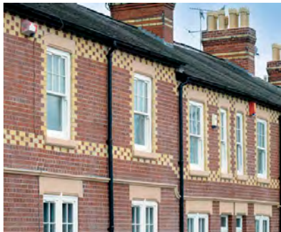
Figure 1.7: Recently restored terraced houses in Knutton with red brick, buff brick banding, sandstone sills, lintels and quoins and blue clay tiles
