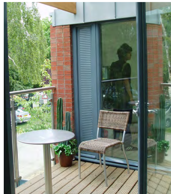
Figure 7.23: A good example of providing private amenity space in the form of a balcony
