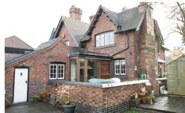
Figure 7.27: Longton Road, Trentham, a successful example of the use of contrasting materials and details on an extension to a listed building
