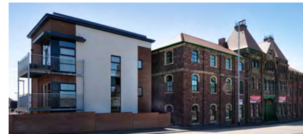
Figure 7.4: Lock 38, new housing which exploits the site's historic features, converting the historic factory frontage for housing with linked new build to define the street space
