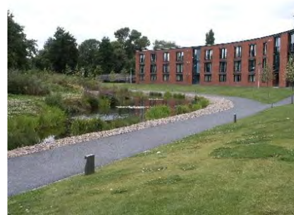
Figure 2.12: Jubilee Campus, Nottingham - University buildings in a 'green' landscape setting based around a lake and wetlands, which also manage surface water run-off and contribute to cooling of the buildings
