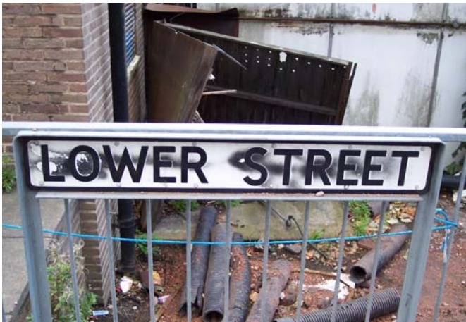
Derelict building frontage
