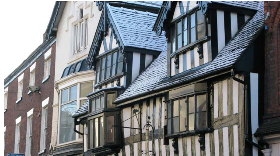
Striking variety in façades on Bridge Street. This is part of the setting for any redevelopment around Ryecroft. © SueC
