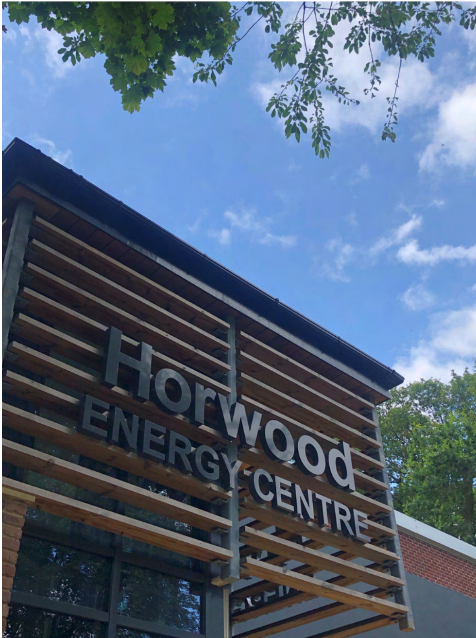
Figure 23 Horwood Energy Centre, Keele University Campus
