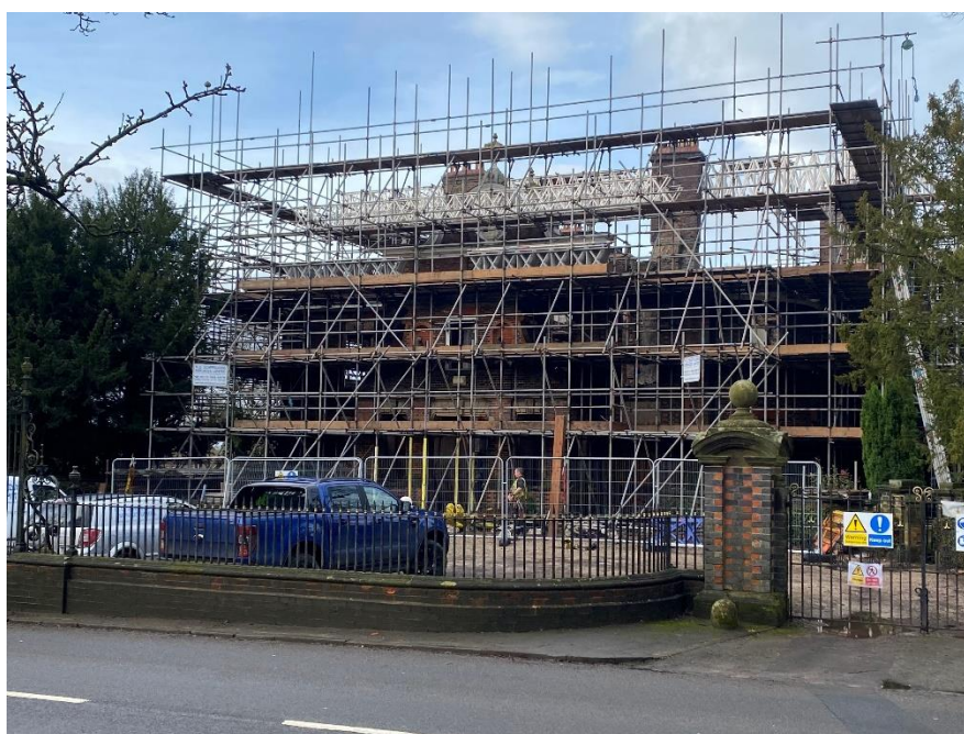
Betley Court scaffolding, January 2021
